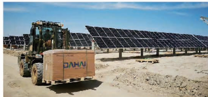
Laiwu Jinneng power station project 13MW
